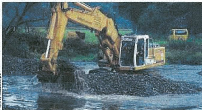
Loosening gravel banks in the R. Sieg
